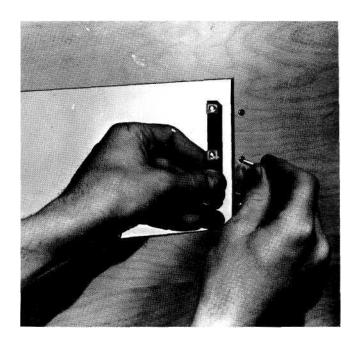
Attach the mounting brackets to the cabinet panel using four screws.
